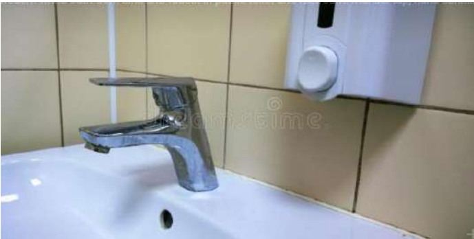
Soap spill on slab and unhygienic
