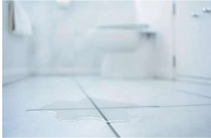
Water spill on floor
